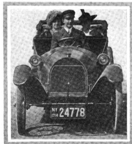
Two views of the new Twombly taxicab to sell for $600. The passengers have an unobstructed view because the driver sits in the center
